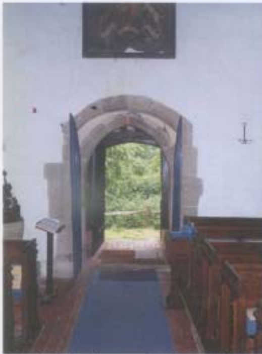
▲ Fig. 10: West doorway of c.1310 with plain pointed arch and segmental rear-arch.
