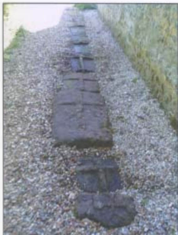
◀ Fig. 41: The line of slabs in the gravel path in front of the north wall of Chithurst church, seen from the west. (Tony and Lesley Voice)
