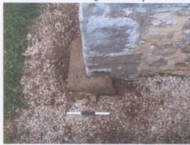
▲ Figs. 13 and 14: Large shaped slabs found as footings on (left) the south-east corner of the chancel and (right), the south-west corner of the nave. They both appear to be coeval with the original eleventh-century structure.
