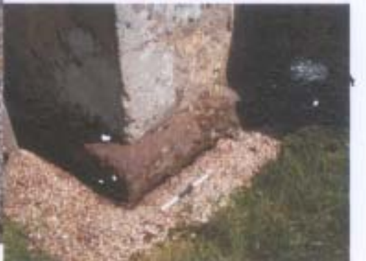
▲ Figs. 13 and 14: Large shaped slabs found as footings on (left) the south-east corner of the chancel and (right), the south-west corner of the nave. They both appear to be coeval with the original eleventh-century structure.
