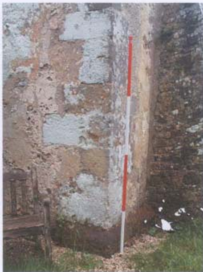
► Fig.18: Rough quoins of c.1310 as a repair to the south west corner (Robert Hutchinson)
