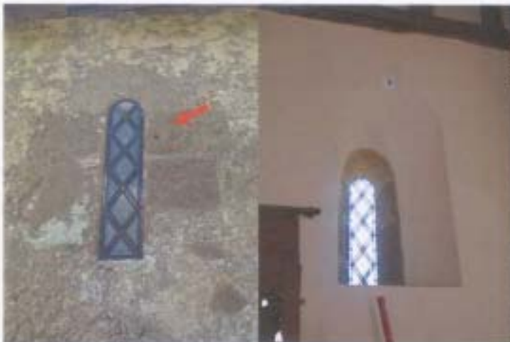
▲ Fig. 7: Exterior and Interior photographs of original unglazed window of c.1080 in north wall of chancel. Note wall thickness, (which averages 0.62 metres throughout the church) as displayed by the interior splay, and the hole on the right of the exterior window which may indicate a bracket for an outside shutter.
