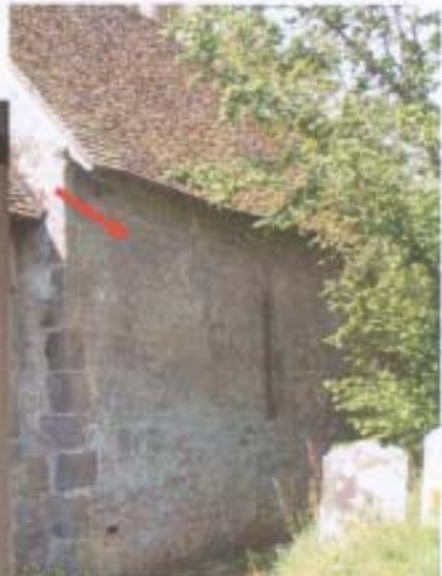
▲ Fig. 7: Exterior and Interior photographs of original unglazed window of c.1080 in north wall of chancel. Note wall thickness, (which averages 0.62 metres throughout the church) as displayed by the interior splay, and the hole on the right of the exterior window which may indicate a bracket for an outside shutter.
