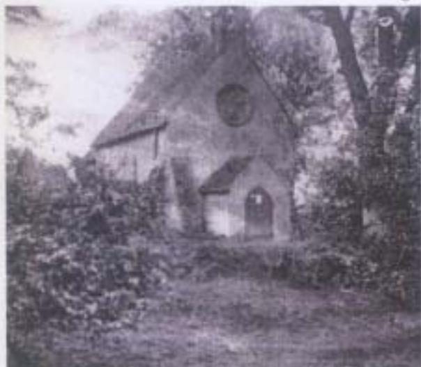
▲ Fig. 15: Photograph of west end of Chithurst church before 1911, showing now removed circular rose window from Iping church and raked buttress on west wall. (via Tony and Lesley Voice).
