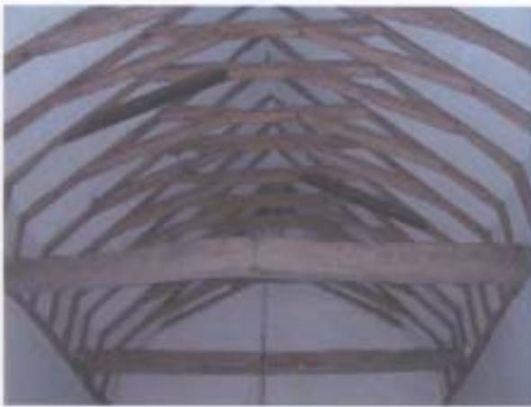
► Fig. 12: Nave roof, looking west, showing exposed trussed rafters and tie-beams.
