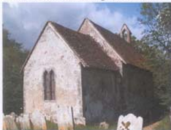
◀ Fig. 2: Chithurst church from the north-east, showing its two celled structure. The east window, with two ogee trefoil lights, was inserted c.1310.
